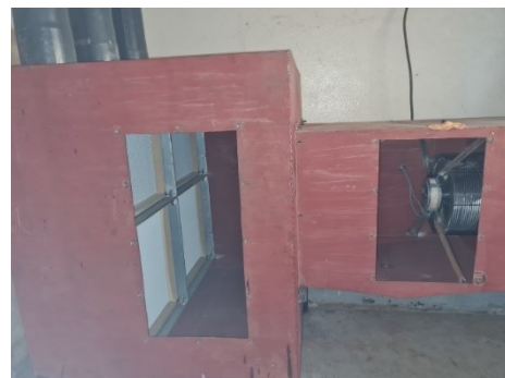
Figure 4: Air system box, with open maintenance doors; H13 filters and radial ventilator visible
