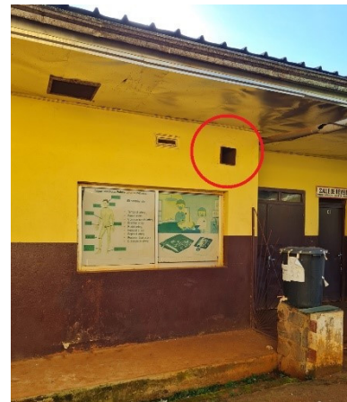
Figure 2: Outside fresh air collector (red circle)
